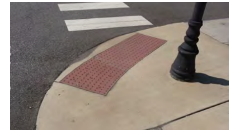
Traffic light pole in front of curb ramp
