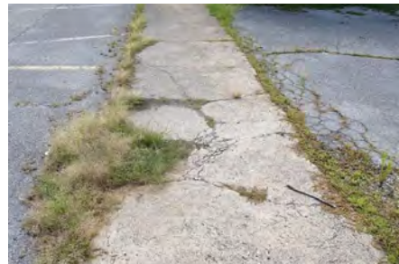
Cracks and grass in walkway
