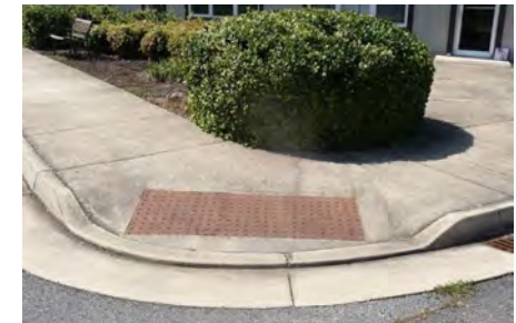
Curb ramp obstructs walkway, not ADA accessible
