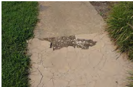
Hole in concrete walkway
