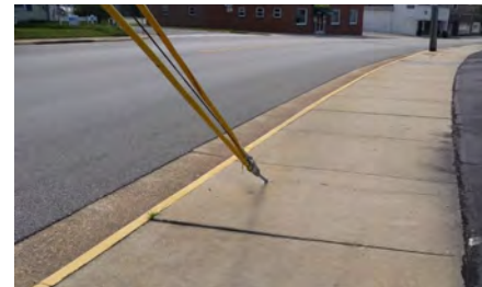
Utility pole cable in walkway
