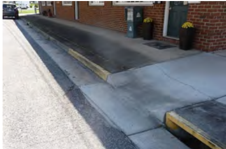
Curb ramp obstructs walkway, not ADA accessible
