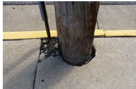
Gap around utility pole, busted concrete
