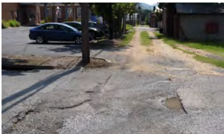
Holes, uneven areas and loose gravel in road, inconsistency in paving material with asphalt turning to gravel
