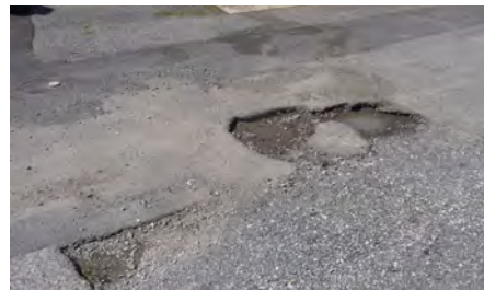
Large pothole in asphalt road
