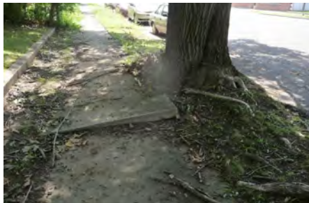
Walkway heaving and damaged from tree roots
