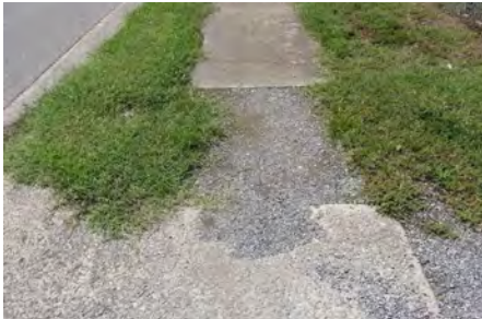
Concrete section missing in walkway
