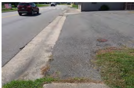
Asphalt from adjacent parking displaces concrete walkway
